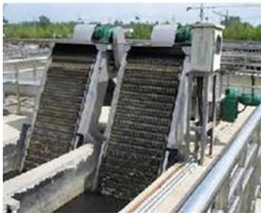
Gambar 2. 3 Mechanical Bar Screen
