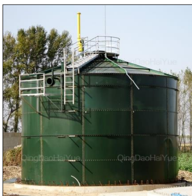
Gambar 2.25 Reservoir Tanki Baja
