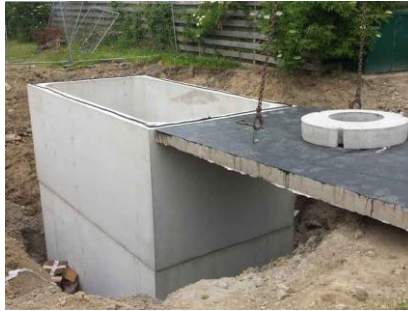
Gambar 2.26 Reservoir Beton Cor
