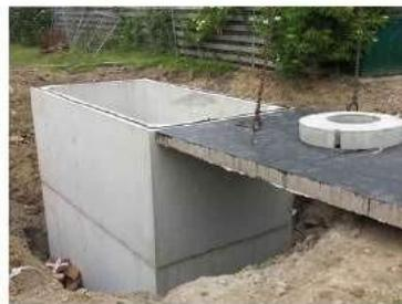
**Gambar 2 . 14** Reservoir Beton Cor
