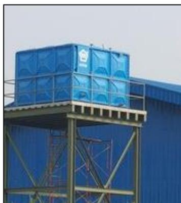
**Gambar 2.23** Reservoir *Fiberglass*
