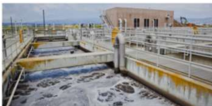
Gambar 2.12 Aerated Activated Sludge
