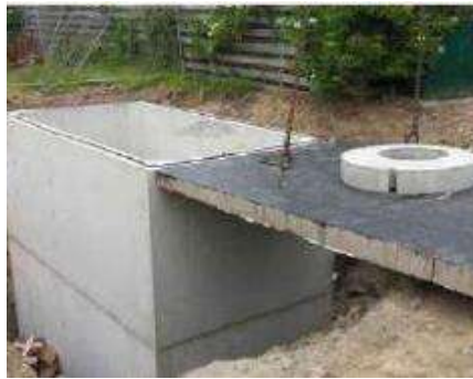
Gambar 2. 22 Reservoir Beton Cor
