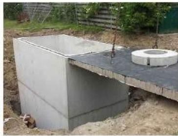
Gambar 2.17 Reservoir Beton Cor
