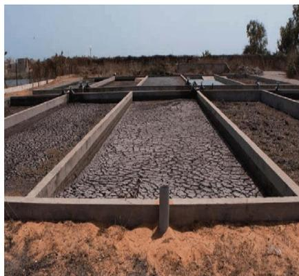
**Gambar 2.17** Sludge Drying Bed
