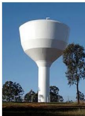
Gambar 2. 18 Reservoir Menara Sumber: BPSDM PU
