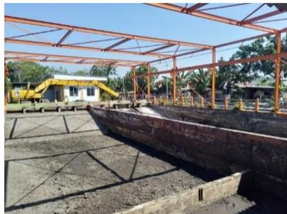
Gambar 2. 3 Unit Solid Separation Chamber di IPLT Keputih
