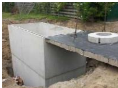
Gambar 2.25 Reservoir Beton Cor
