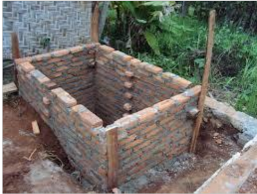
Gambar 2. 29 Reservoir Pasangan Bata
