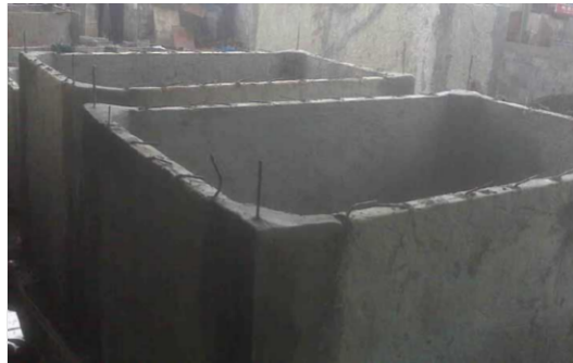
Gambar 2. 28 Reservoir Beton Cor
