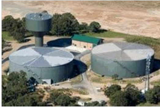
Gambar 2. 27 Reservoir Tangki Baja
