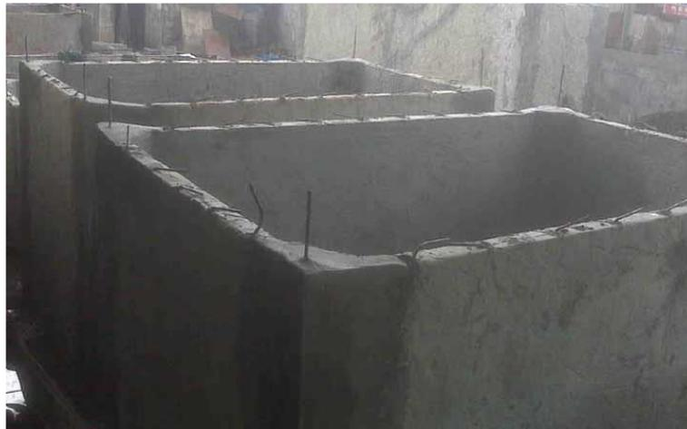
Gambar 2.13 Reservoir Beton Cor
