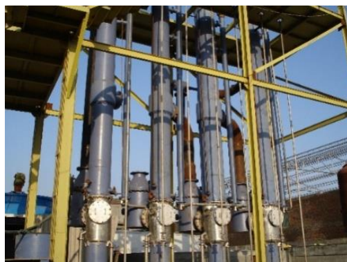
Gambar 3. 8 Falling Film Evaporator
