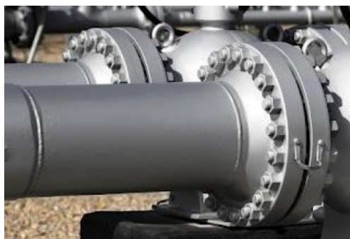
GAMBAR 2. 178 FLANGE PIPA
