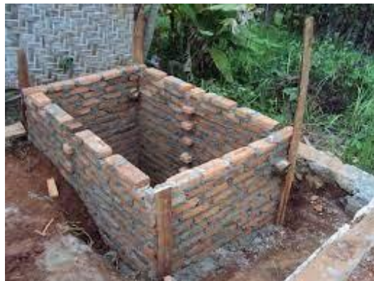
GAMBAR 2. 22 RESERVOIR PASANGAN BATA
