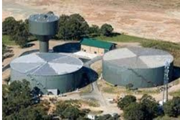
GAMBAR 2. 159 RESERVOIR TANKI BAJA
