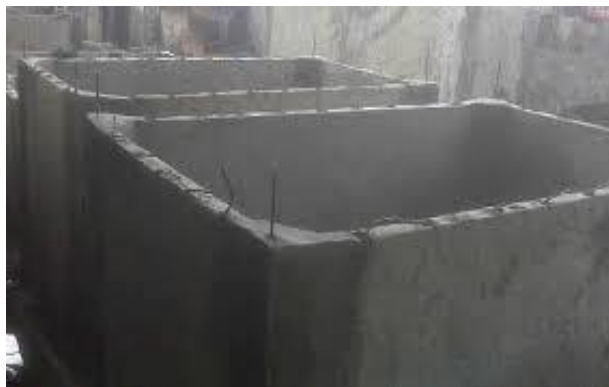
GAMBAR 2. 20 RESERVOIR BETON COR
