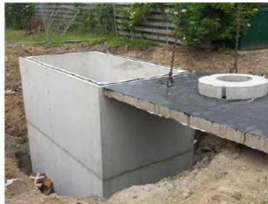
Gambar 2. 28 Reservoir Beton Cor
