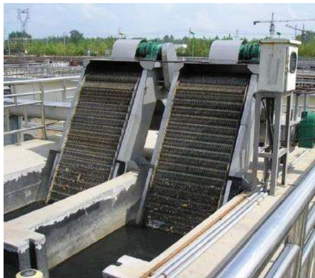
Gambar 2.3 Mechanical Bar Screen
