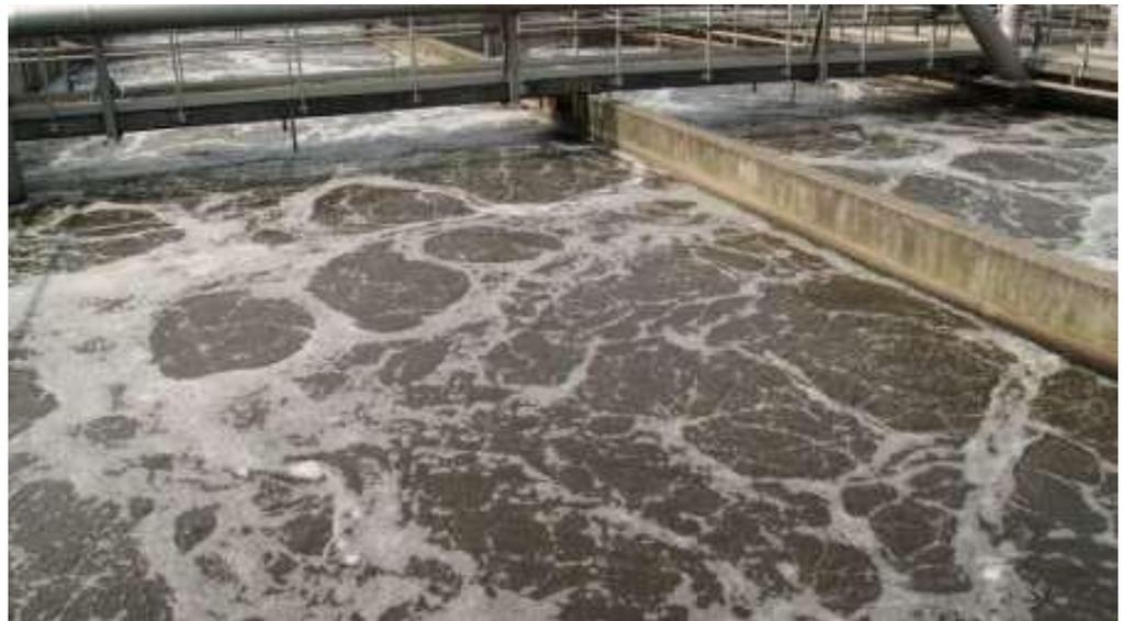
Gambar 2.15. Aerated Activated Sludge
