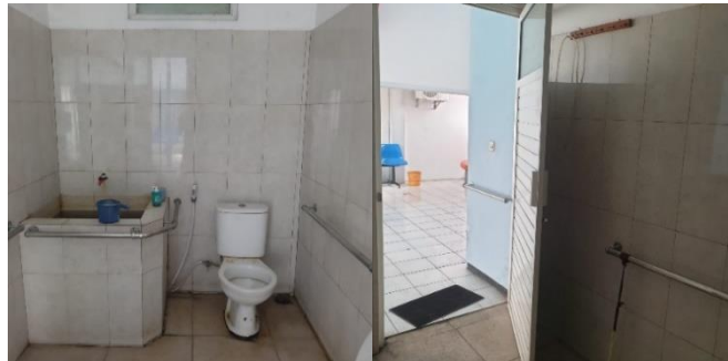
Gambar 2. 45 Toilet YPAC Surabaya
