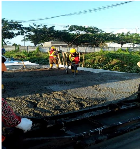
Gambar 3.16 Proses Vibrasi
