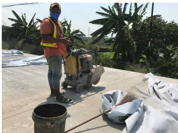
Gambar 3.7 Proses Cutting
