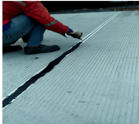
Gambar 3.9 Proses Joint Sealant
