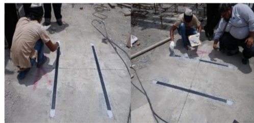
Figure 20. CFRP installation process
