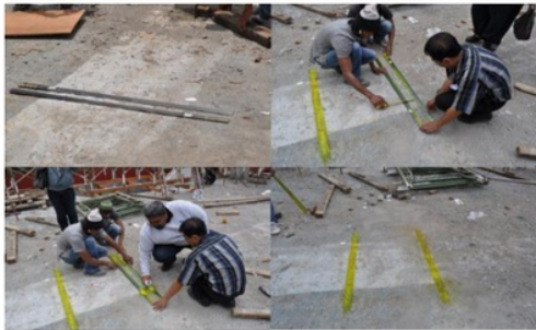
Figure 19. Implementation of Measurement and concrete surface markings
