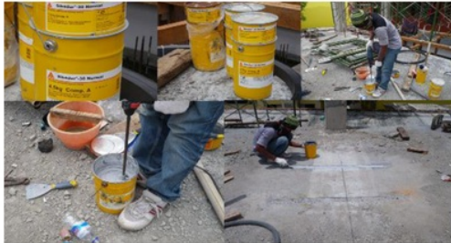
Figure 21. The mixer process and installation of CFRP species
