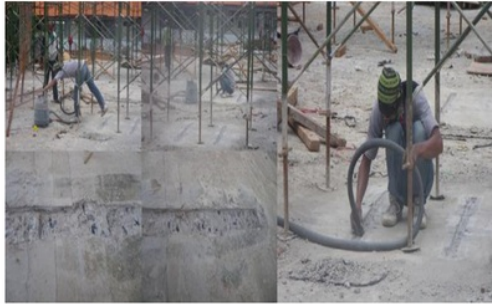
Figure 18. Implementation process and results Patching
