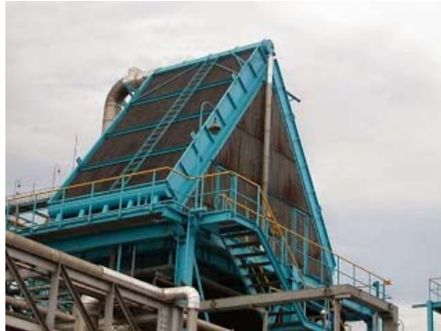
Gambar II.2 Air Cooled Condenser
