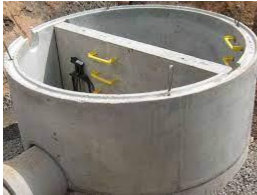
Gambar 2. 26 Reservoir Beton Cor
