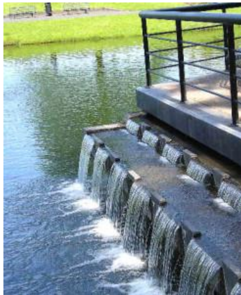
Gambar 2. 11 Multiple Tray Aerator
