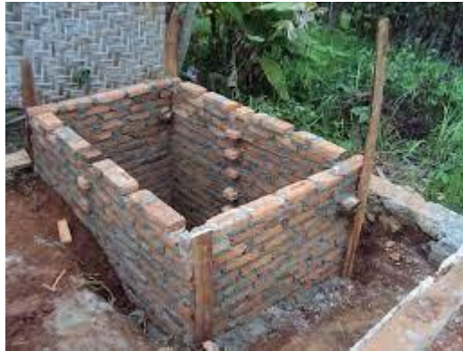
Gambar 2. 27 Reservoir Pasangan Bata
