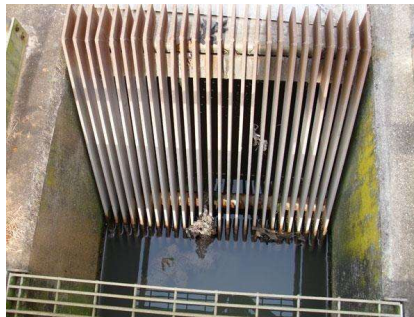
Gambar 2. 4 Manual Bar Screen
