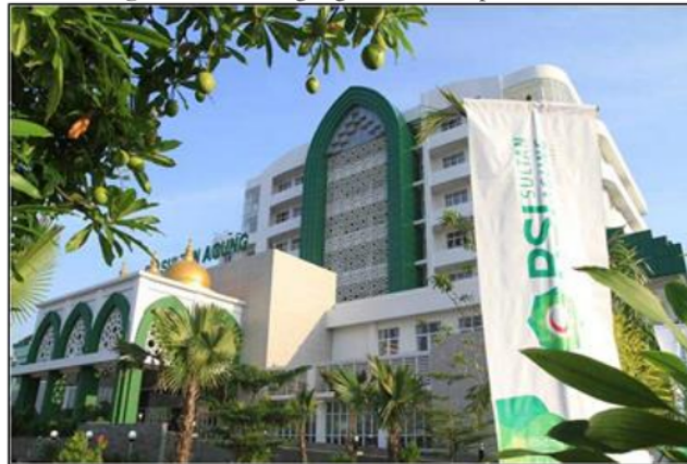
Figure 2 Sultan Agung Islamic Hospital
