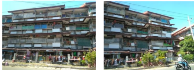
Figure 3. Penjaringan Sari I flats facade Surabaya
